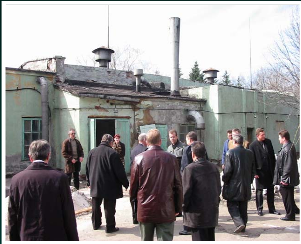
Process building external
